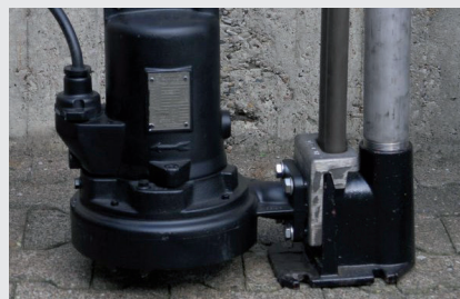
| Couple the pump to the guide rail
