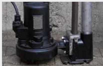
| Couple the pump to the guide rail
